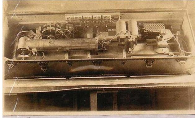
Rare picture of Fessenden's radio telephone (HF generator) apparatus of 1907
